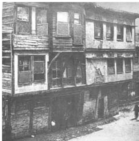
Figure 7. The examples of traditional houses with wood clapboards and " hımış " at the beginning of the 19th century in Istanbul (Eldem,1984).
