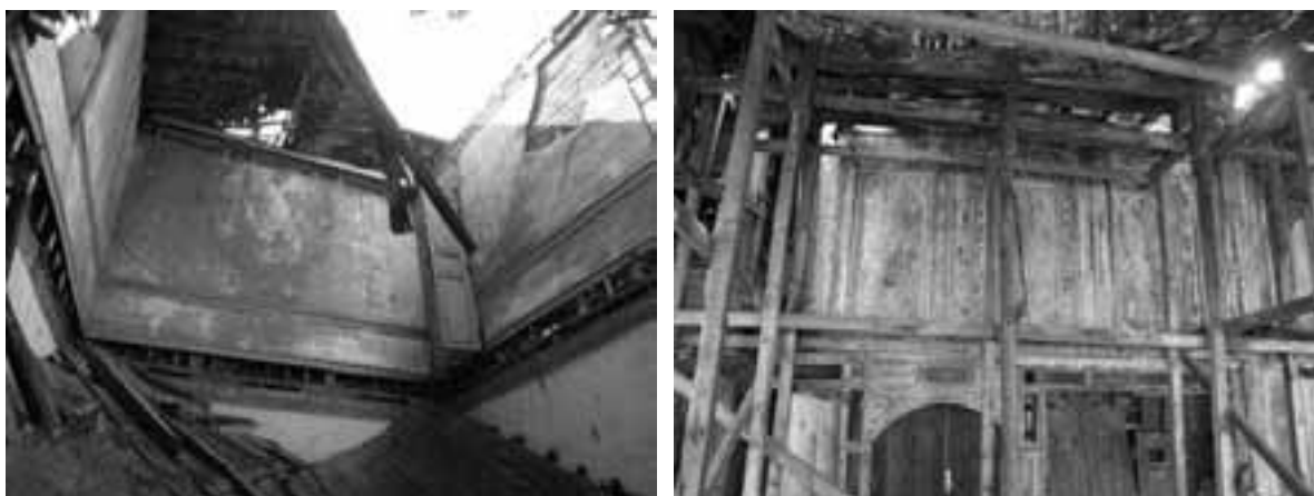
Figure 8. Lack of maintenance: case of Amcazade Yali on Bosphorus (Can Binan’s archives).
