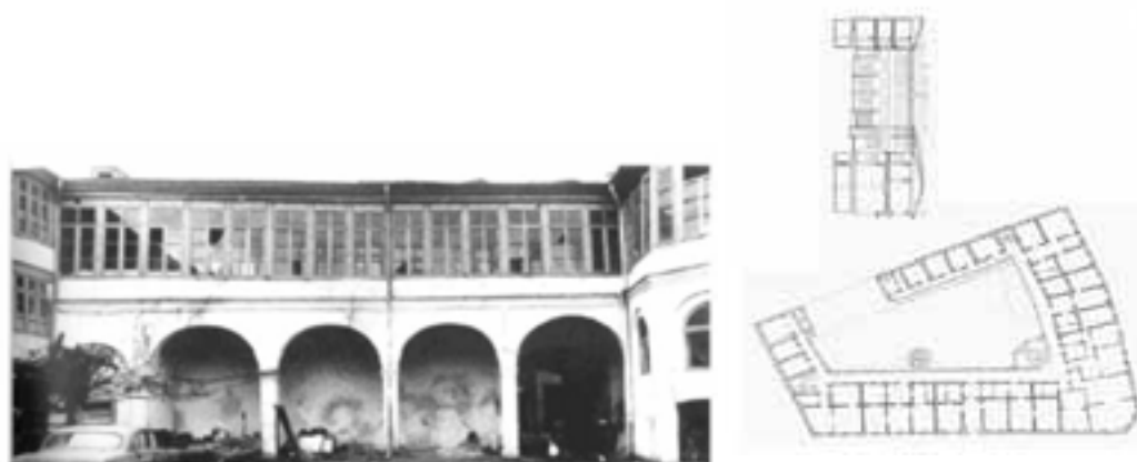
Figure 6. The "Patria" Inn, Bucharest – facade and sidewalls (Joja C-tin., 1999a).
