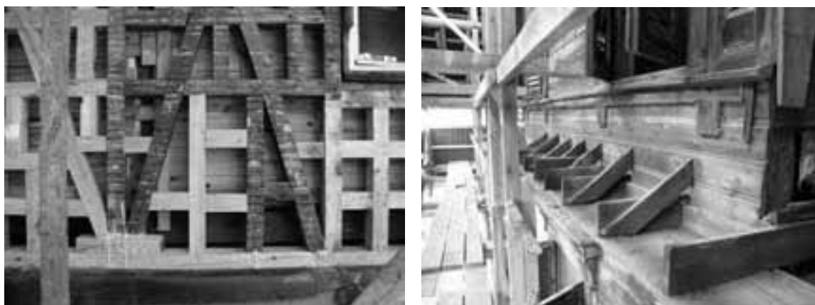
Figure 11. Interior and exterior bracing systems (Can Binan's archives).
