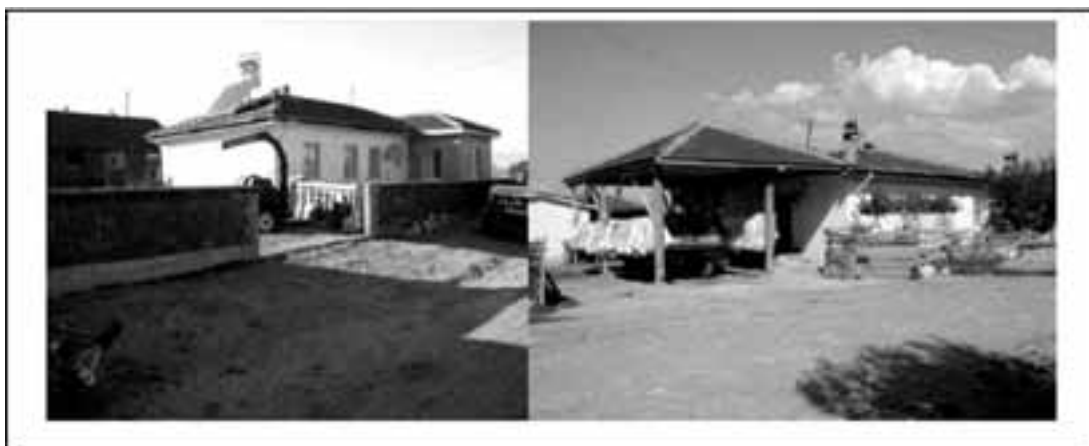
Figure 4. Additional parts of post-disaster houses in villages of Dinar.
