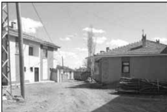
Figure 3. Buguoren Village (PDH were constructed in the existing settlement).
