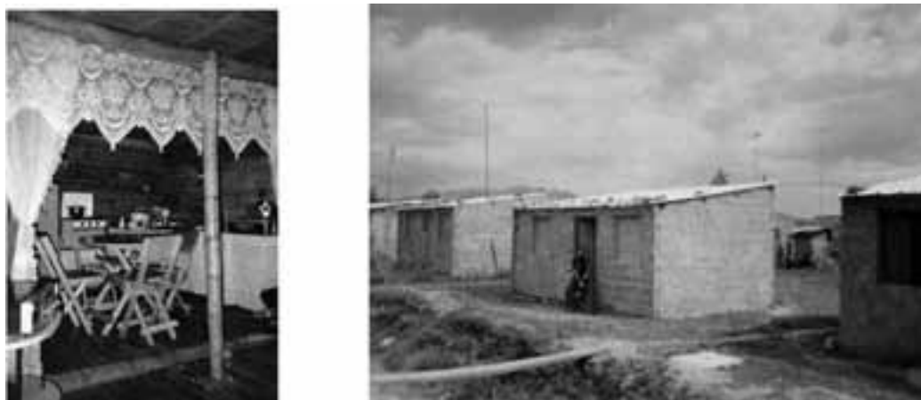
Figure 1. Left : Interior of a spontaneous unit in Armenia, Colombia. Despite that the unit is built on illegally occupied land, the interior demonstrates the care for comfort and quality of space. Right : unit in Choluteca, Honduras. The design dramatically separates indoor and outdoor space creating “the box-effect”.
