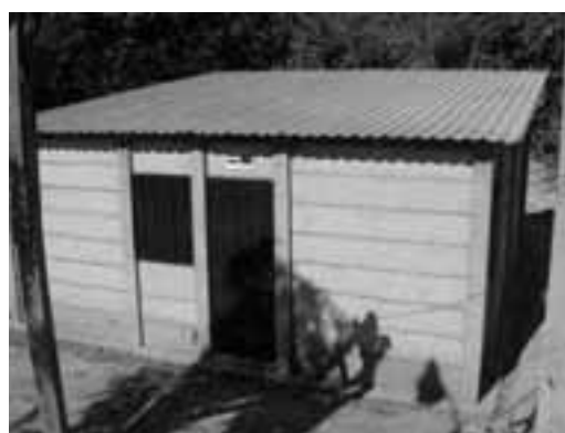
Figure 2. RC Prefabricated house
