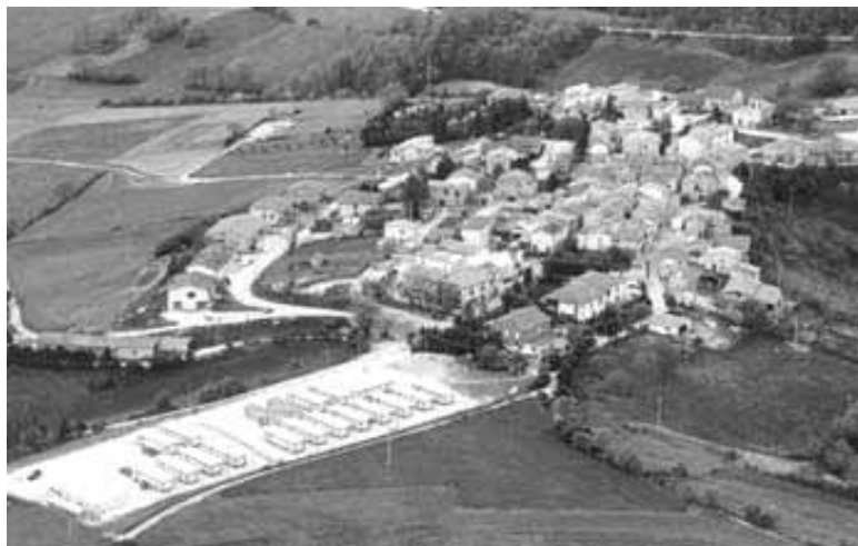
Figure 1. Example of emergency settlement system in Umbria for post-disaster reconstruction (località Forcatura – Foligno).
