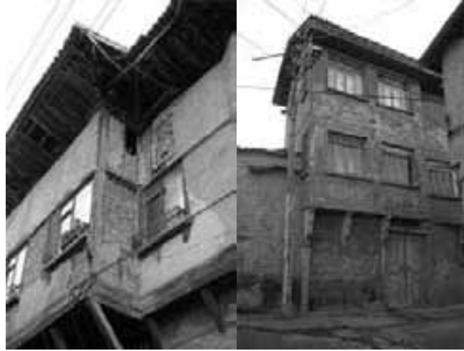
Figure 2. Examples of traditional houses that openings and construction systems have changed.
