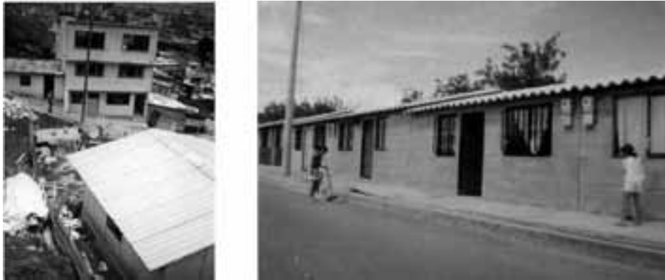
Figure 2. Left : Informal settlement in Bogotá showing 4 different stages in the housing evolution process: from a shack made of scrap wood to a three storey unit made of concrete and masonry. Right : 1-storey units in El Cantarito. Despite that higher densities were obtained and infrastructure was provided, few months after the project was finished, users had already modified the rigorously standardized facades to personalize them with colours and finishes.
