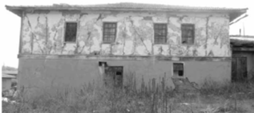
Figure 2. A building in Yuva Village, Cankiri Province, Turkey (Dikmen 2005), which withstood an earthquake of magnitude 5.9 on Richter Scale 06-06-2000.
