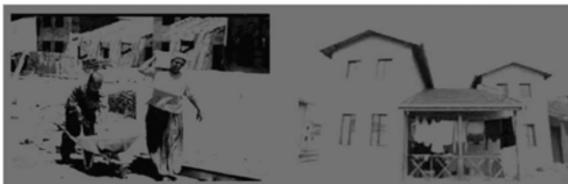
Figures 11 and 12. Public participation in the construction of new houses.
