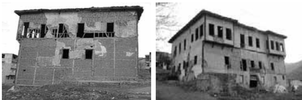
Figure 4. The timber frame with adobe infill construction in Osmaneli.
