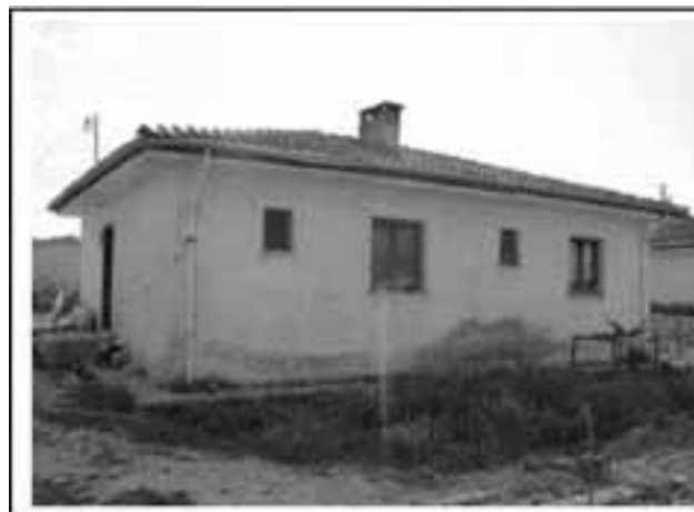
Figure 3. Post-disaster houses in villages of Dinar.
