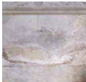
Distacco intonaco interno. Detachment of interior plasterwork.
