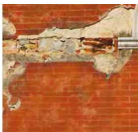
Distacco e lacuna elemento marmoreo. Detachment and gap in the marble element.
