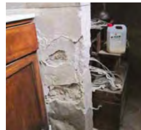
Distacco e rigonfiamento intonaco interno. Detachment and swelling of interior plasterwork.
