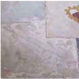
↑ Esfoliazine ed efflorescenze dei pavimenti marmorei interni. Exfoliation and efflorescence on interior marble floors.
