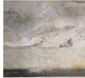
Efflorescenze intonaci interni. Efflorescence on interior plasterwork.
