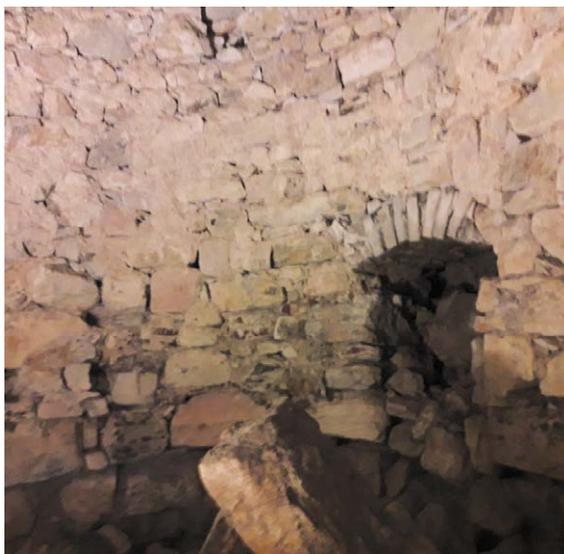
Figure 6 – Underground room at *limonaia* Fondo Campagnola (Gargnano) to collect and drain the water springing from the rocks.
