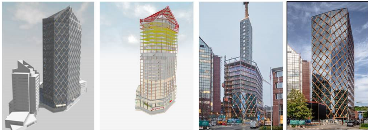
Fig. 10: The Kinum project; BIM, structural-only BIM, construction, completed building (left to right).
