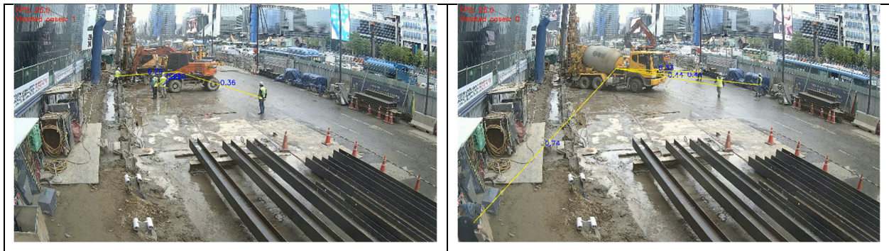
Figure 4. Distance estimation using depth estimation and object detection.
