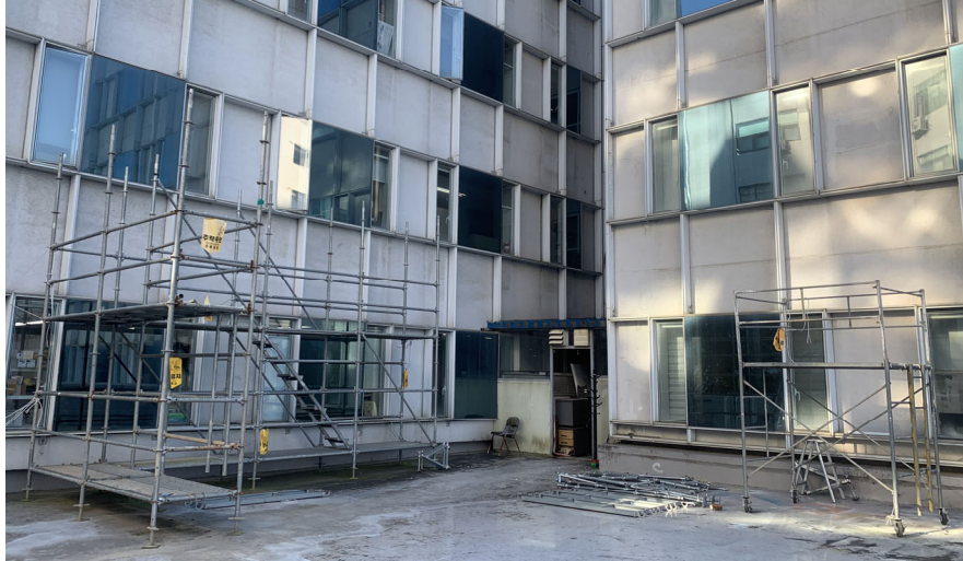
Fig. 3: The construction jobsite using both fixed and mobile scaffolding
