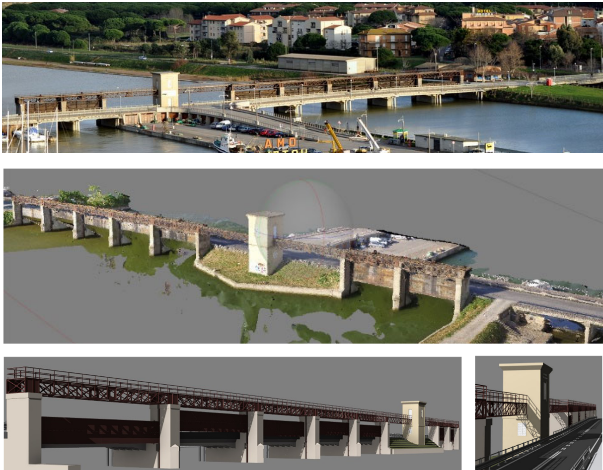
Fig. 5, 6, 7: View of Giorgini Bridge | Digital photogrammetry from drone | Views of the BrIM model
