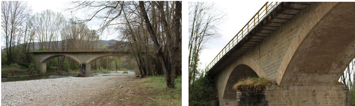
Fig. 11, 12: Views of Toppoli Bridge over the Arno River
