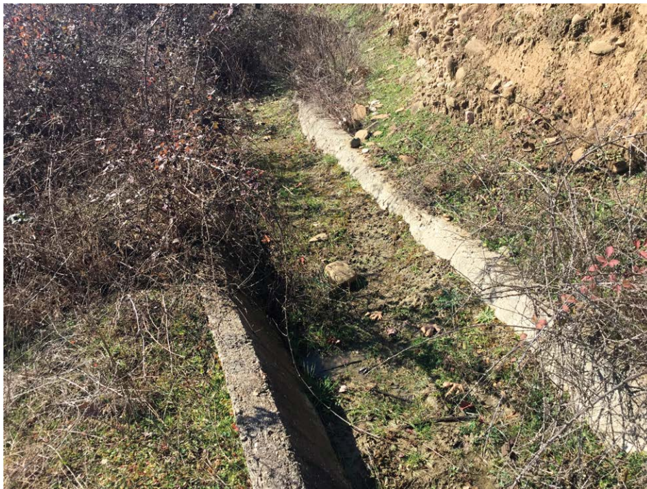
Figure 5.7 – A section of disused hydraulic- agricultural canalisation in the alluvial terraces on the hydrographical right of the Lëngarica.
