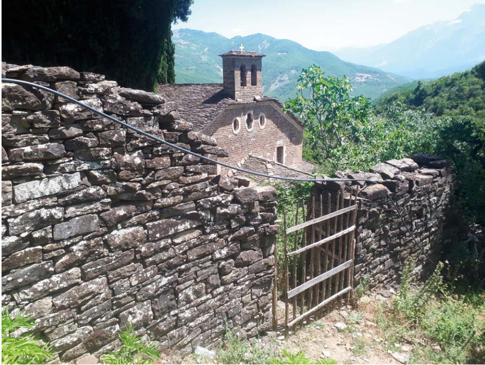
Figure 2.40 – Detail of the cemetery enclosure wall.
