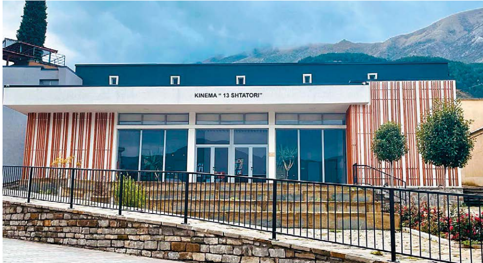
Figure 1.29 – The recently renovated cinema in Përmet.
