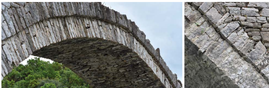
Figure 3.38 – Kadiu Bridge, details of the stone archivolts.
