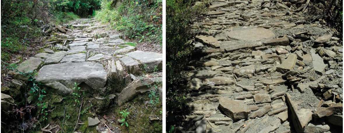
Figure 3.31 – Details of the laying of the kalldrēm .
