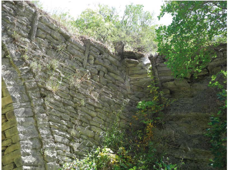
Figure 3.41 – Bënjë Bridge, the masonry joined by vertical stone elements, connected to a section of wall on overhanging slabs.
