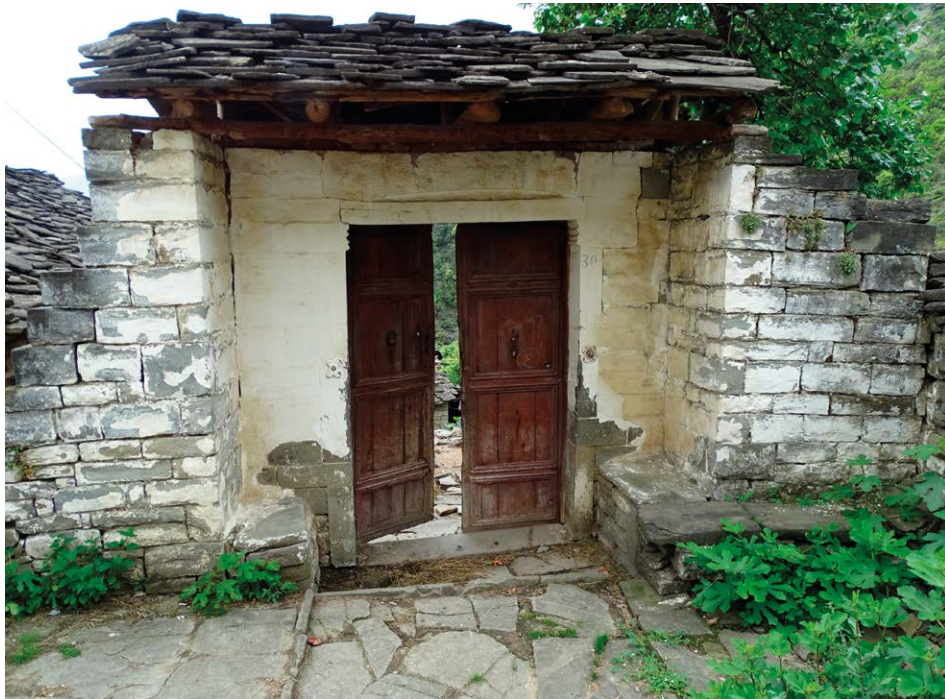
Figure 2.35 – Entrance to the courtyard of a village house with the traditional sofat .
