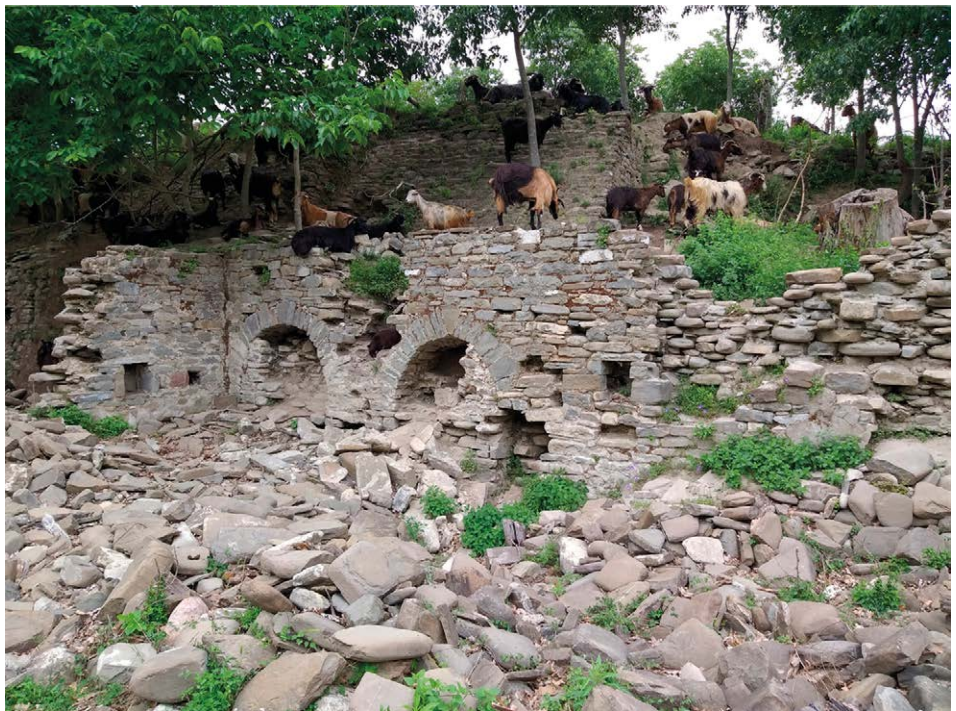
Figure 2.6 – The ruins of the old Bënjë Mill.
