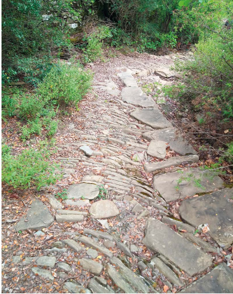
Figure 3.32 – Section in kalldrëm with the edges blocked by large slabs.
