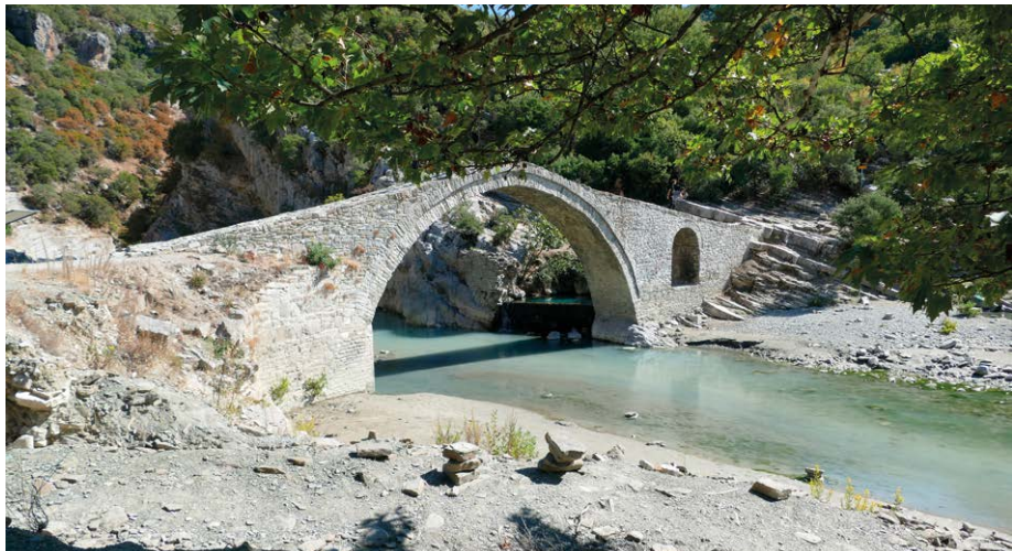
Figure 1.21 – The Kadiu Bridge.
