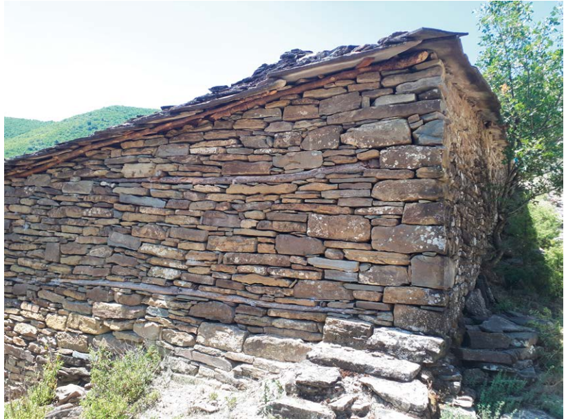
Figure 2.44 – Detail of the load-bearing masonry of an agricultural outbuilding.
