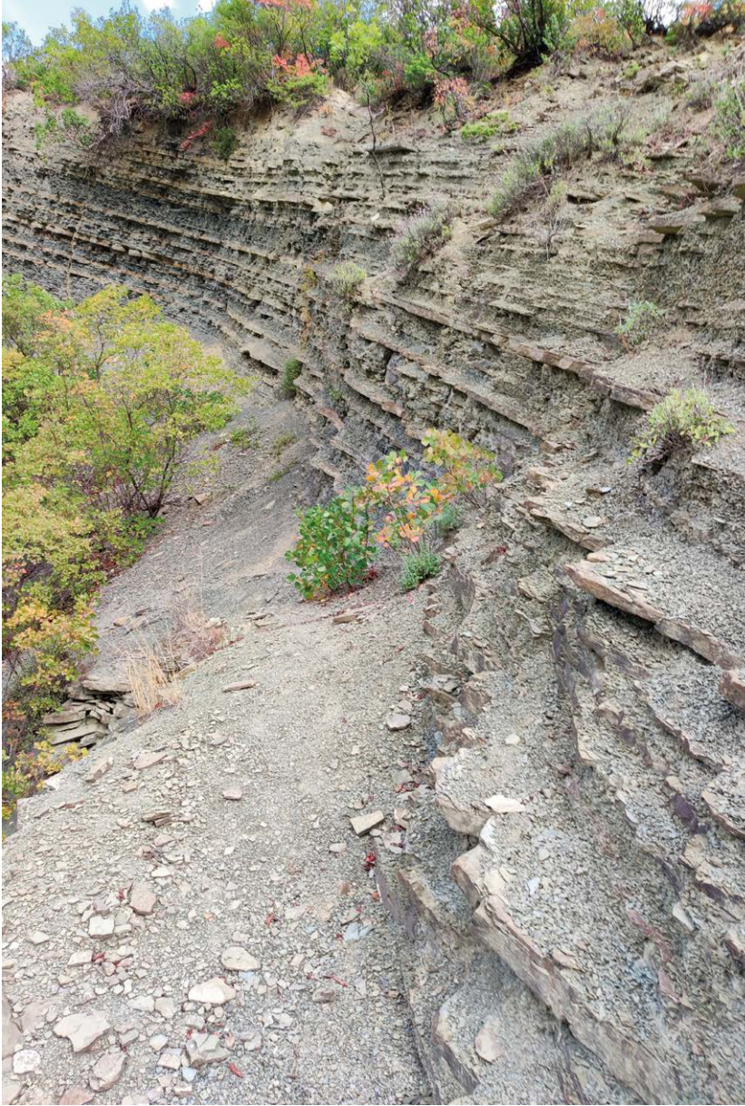
Figure 3.22 – Rock face near Bënjë Bridge.
