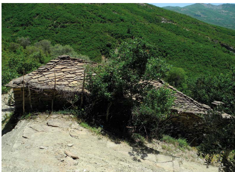
Figure 3.33 – Roofing of a building made of the same slabstone used for the path.
