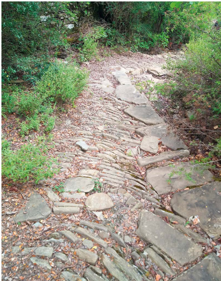
Figure 3.32 – Section in kalldrēm with the edges blocked by large slabs.
