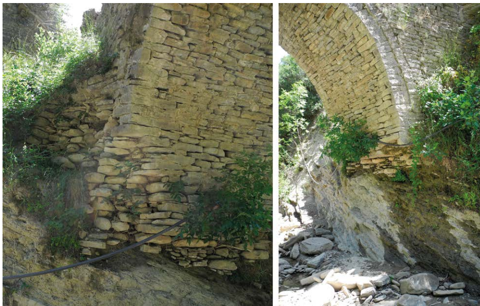
Figure 3.43 – Details of the left abutment of the Bënjë Bridge.
