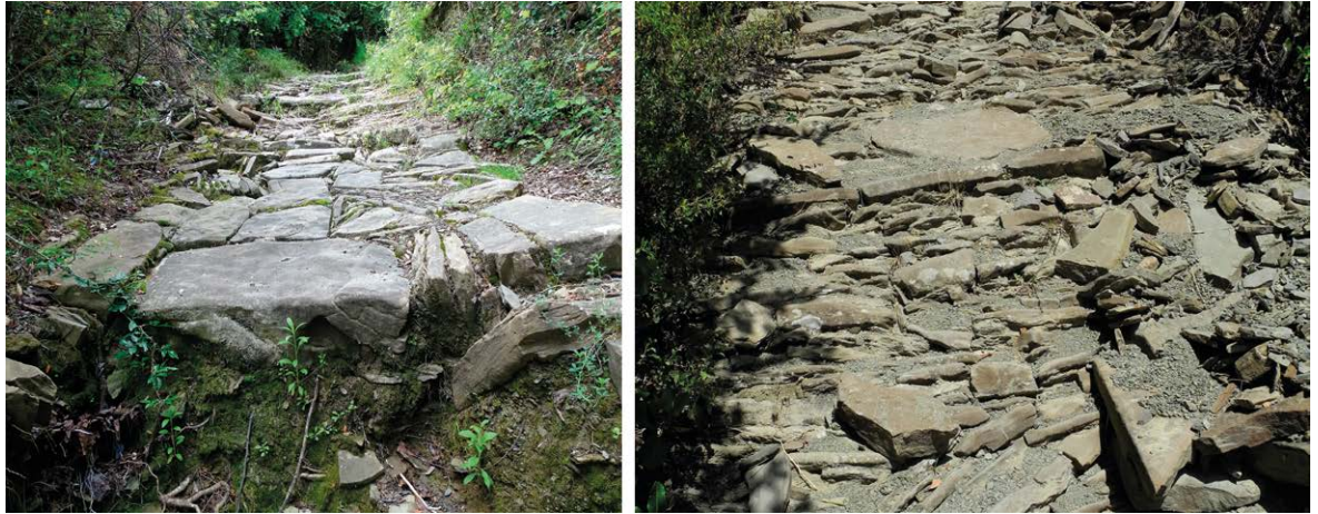
Figure 3.31 – Details of the laying of the kalldrēm .
