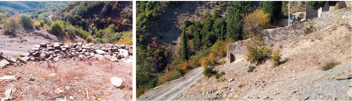
Figure 4.42 – State of deterioration of the walls supporting the terracing. Table 4.12 – Narrative master plan of Functional Lot 3: Interventions relating to the external areas adjacent to the architectural complex.
