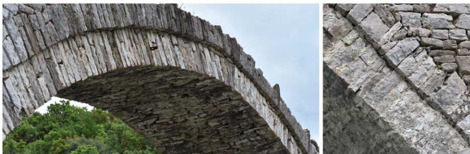
Figure 3.38 – Kadiu Bridge, details of the stone archivolts.
