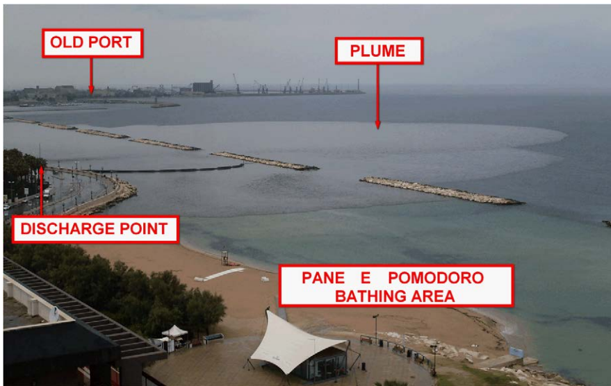
Figure 2 – Turbidity plume recorded on July 24 th from the ARPA Puglia administrative building.
