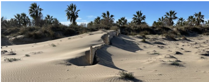
Figure 2 – Sand fences at the Northern campsite almost completely buried by sand, showcasing the natural accumulation process over time.
