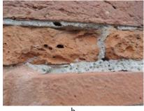
Figure 6 – Forte dei Marmi (a); particular of re-pointed mortar and brick erosion phenomena (b).
