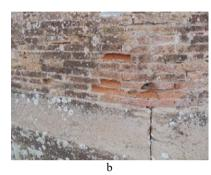
Figure 5 – Forte di Marina di Castagneto (a); particular of biological growth phenomena (lichens) and brick erosion (b).
