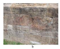
Figure 4 – Forte di Marina di Bibbona (a); particular of exfoliation phenomena caused by improperly installed Pietra Panchina (b).
