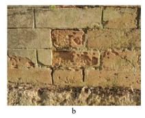
Figure 2 – Forte San Rocco (a); particular of the alveolisation phenomena that have completely eroded the bricks (b).
