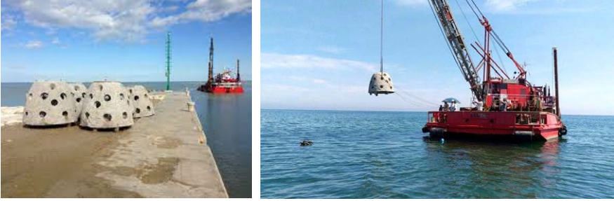
Figures 5 a, b – Positioning of Reef ball.
