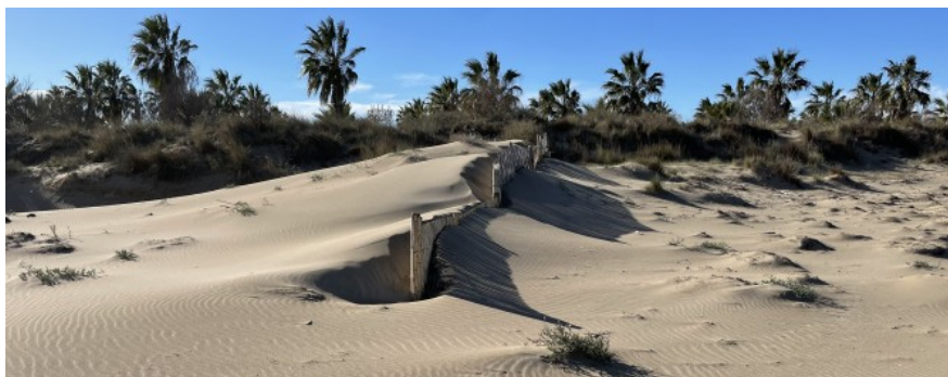
Figure 2 – Sand fences at the Northern campsite almost completely buried by sand, showcasing the natural accumulation process over time.
