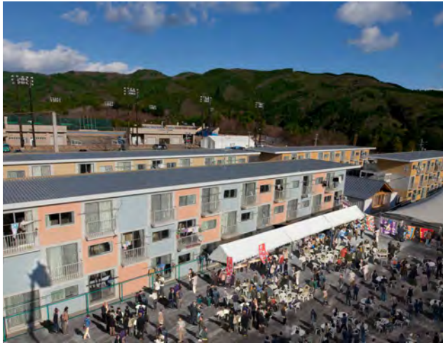
← Market and community center by Shigeru Ban, Onagawa, Japan, 2011.
