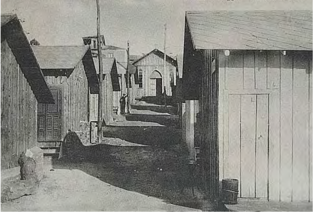
↑ Comitato Milanese temporary district, Reggio Calabria, 1908.
