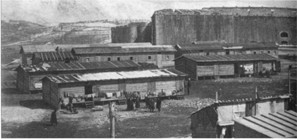
↑ Temporary sheds neighborhood, Parco del Castello, L'Aquila, 1915.
