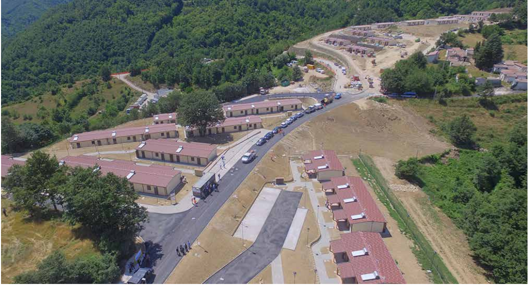
↑ Temporary village of Accumoli under construction, 2017.
