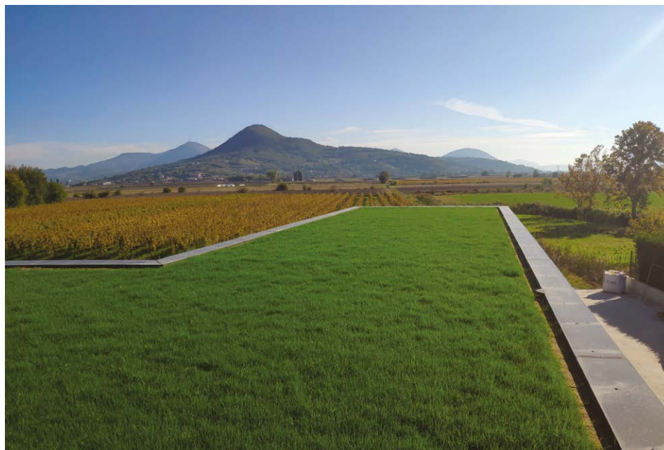
Fig. 6 – Blue-green roof in Nevio Scala Winery in Lozzo (Source: DAKU Italia 2025).
