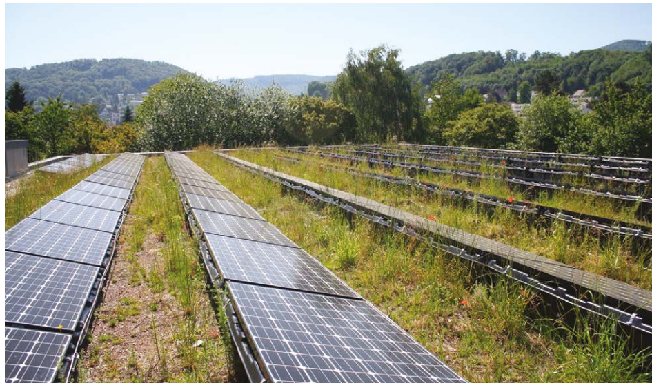
Fig. 5 – Biosolar roof on Hallenbad roof (MuttENZ, Basel) (Source: Catalano 2014).
