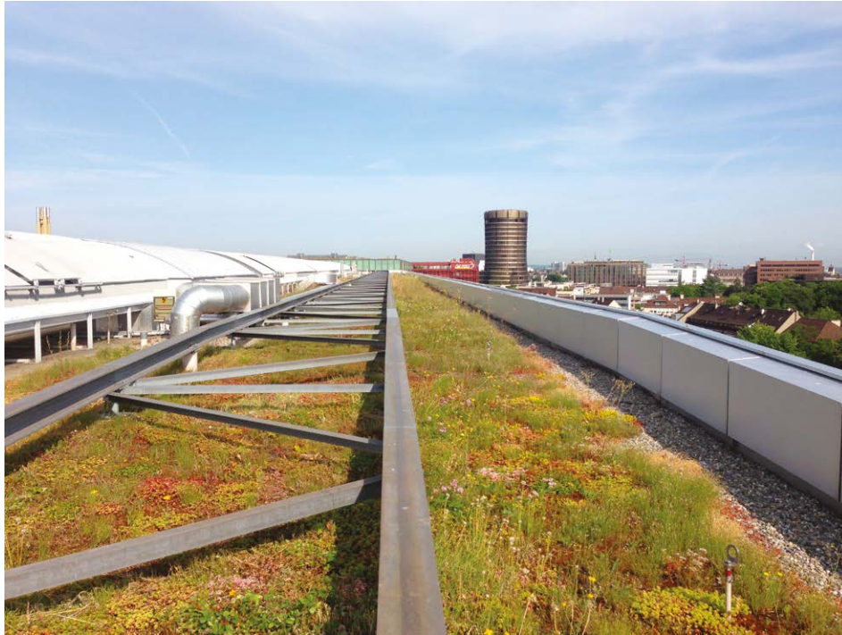
Fig. 1 – Extensive green roof in Basel (Source: Catalano 2013).
