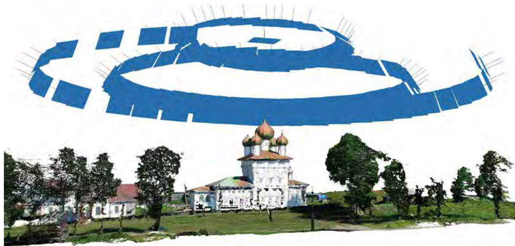
Next page, Fig. 09 Uavs for the definition of punctual database complexes All the monuments had been acquired thanks to a "point of interest" mode set on the drone. The goal is to obtain a better quality data of the building and then integrated these digital output with the general point cloud of the terrain.
