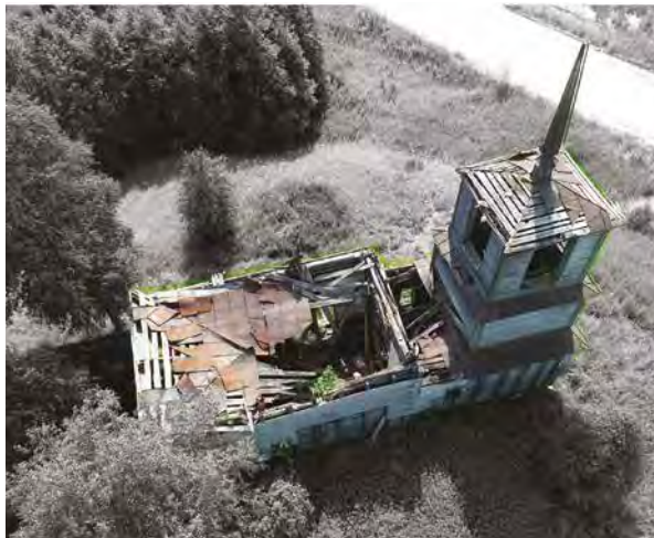
Traditional building abandoned
