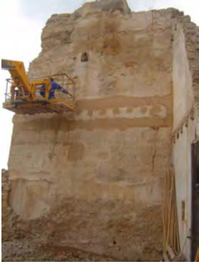
↑ Fig. 12 Consolidation of the Western Wall The west façade of James I's House during consolidation works.
