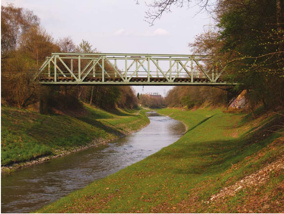
Fig. 2 – Testo Emscher river at Herne and Recklinghausen (Germany). In the background the electricity-museum (Source: Arnoldius 2006, Wiki Common CC By 4.0).
