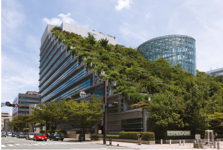
Fig. 9 – Planter green roof in Fukuoka, Japan, designed by Emilio Ambasz (Source: Kenta Mabuchi 2013).
