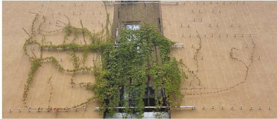
Fig. 7 – Green façade in Budapest at Bastya Park (Source: Hasanaj 2024).
