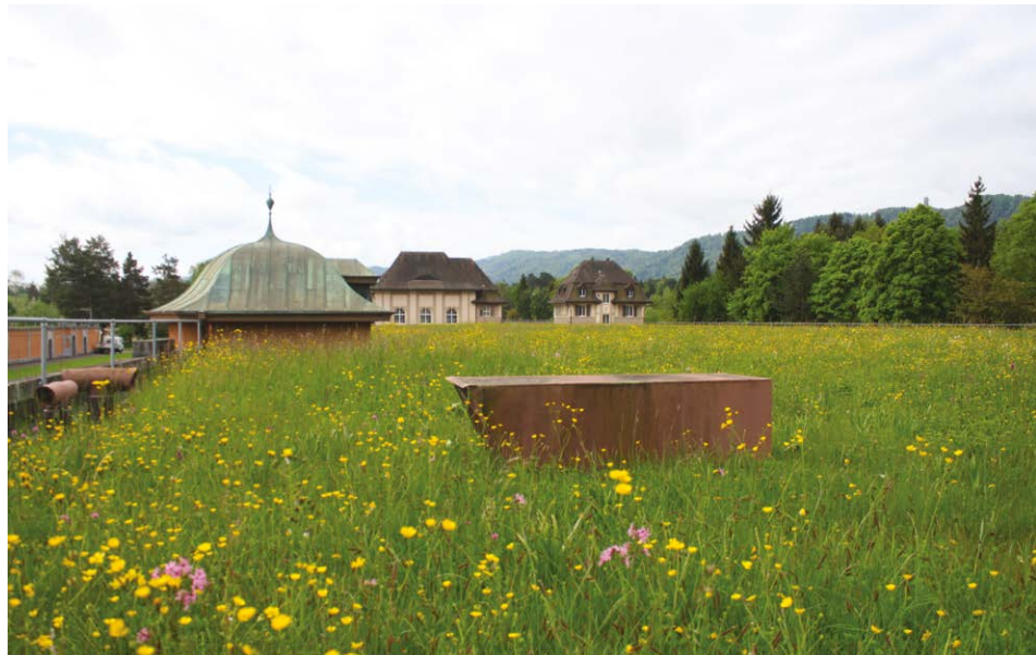
Fig. 3 – Semi-intensive Green Roof of the Water Filtration Plant in Wollishofen, Zurich, Switzerland (Source: Chiara Catalano 2013).
