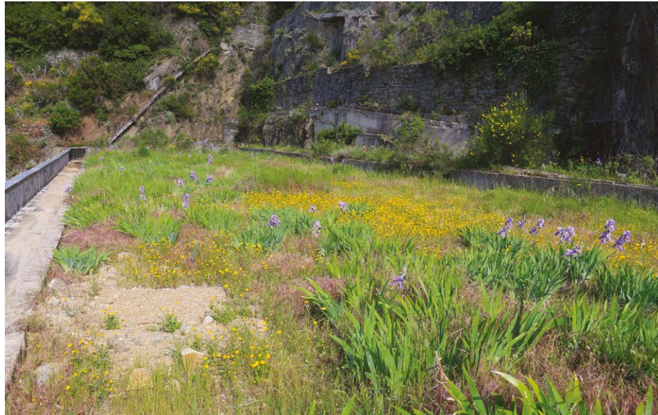
Fig. 4 – Biodiverse roof on a multi-level parking building in Manarola, Liguria, Italy (Source: Riccardo Guarino 2016).
