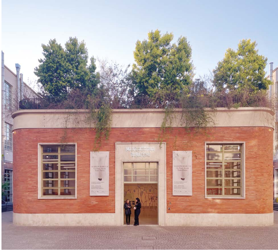
Fig. 2 – Intensive Green Roof at Manifattura Tabacchi in Florence (Source: Hasanaj 2025).
