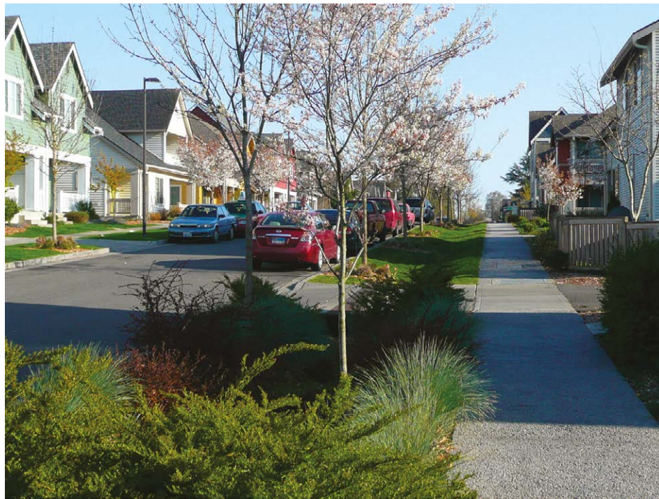
Fig. 6 – Bioswales for treating stormwater runoff from street in Seattle (Source: Architectsea 2011).
