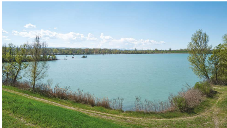
Fig. 1 – Flood mitigation basin of the Secchia River with integrated implementation of vegetation. Basin in Rubiera, Reggio Emilia, Italy.
