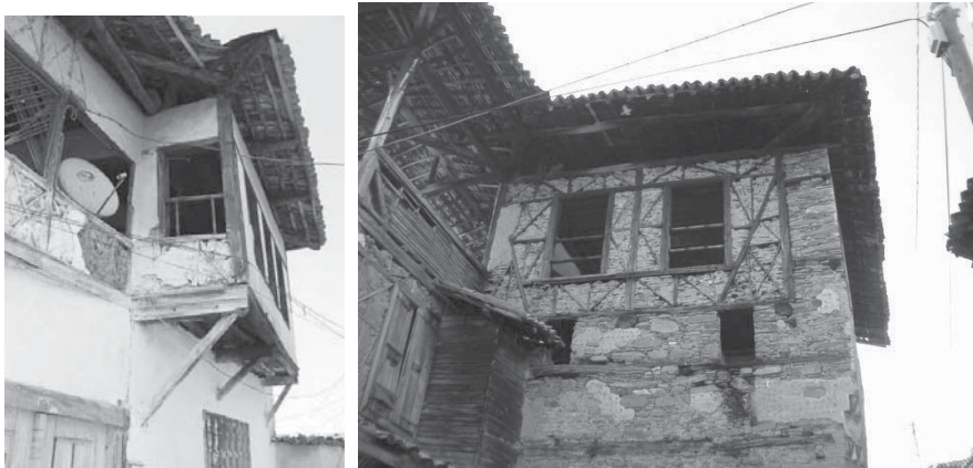
Fig. 4. The timber frame examples from (a) - Kula , (b) – Birgi Houses.
