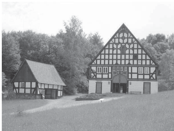
Fig. 1. Westphalian Open Air Museum Detmold; monitoring and control measures since 1999.
