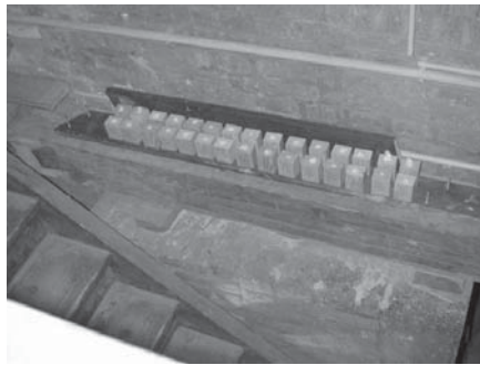
Fig. 6. Control blocks to monitor success (Aachen Cathedral).
