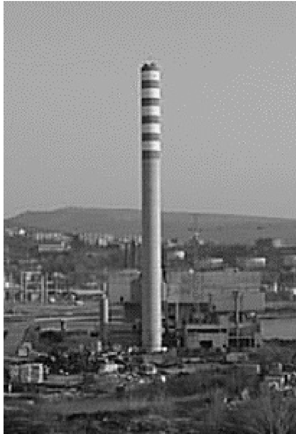
Figure 6.6 Concrete chimney used for in situ experimentation
