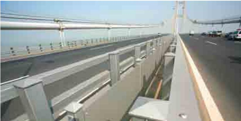
Figure 3: Central stabilizer mounted on the deck of Runyang Bridge
