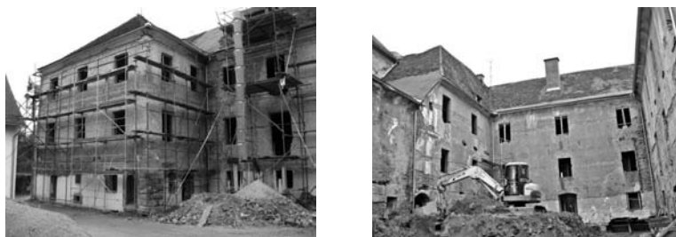
Fig. 1. Views to the east wing (tower) and the western façade of the monastery during a reconstruction.
