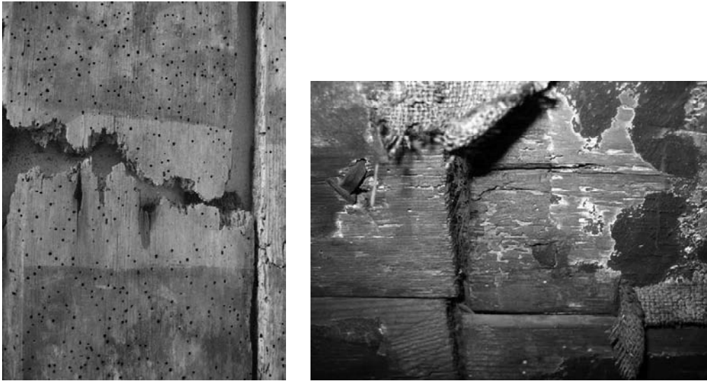
Fig. 5 Anobium punctatum attacks: (a) areas with infiltrations; (b) under interstitial canvases
