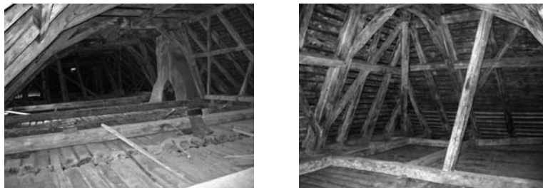
Fig. 3. Typical timber roof beams and massive floors in the attics.
