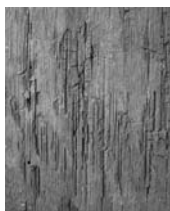
Fig. 5 – Wet rot with cuboidal cracking.
