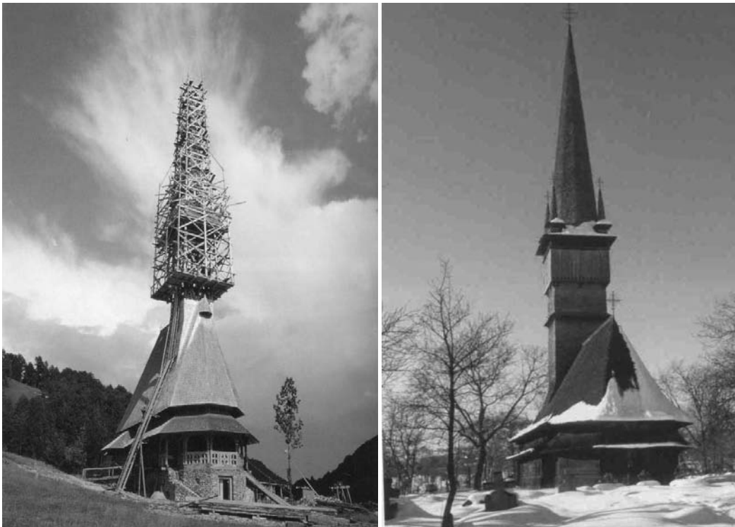
Fig. 3 Maramureș wooden church during and after repair
