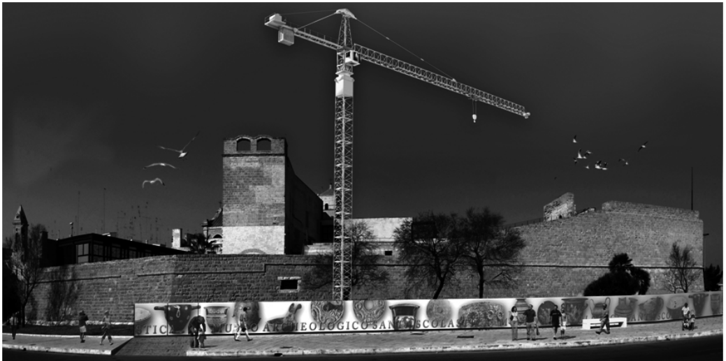
Bari, The archeological Museum of Santa Scolastica. Building site fencing.
