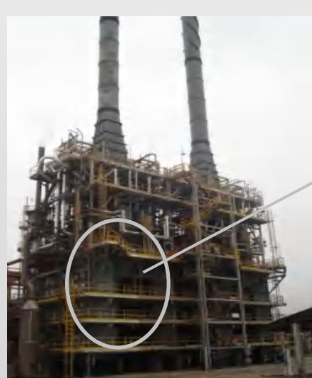
Figure 1. Eihane pyrolysis furnace for the production of ethylene.
