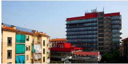
Fig. 2. ATC office building
