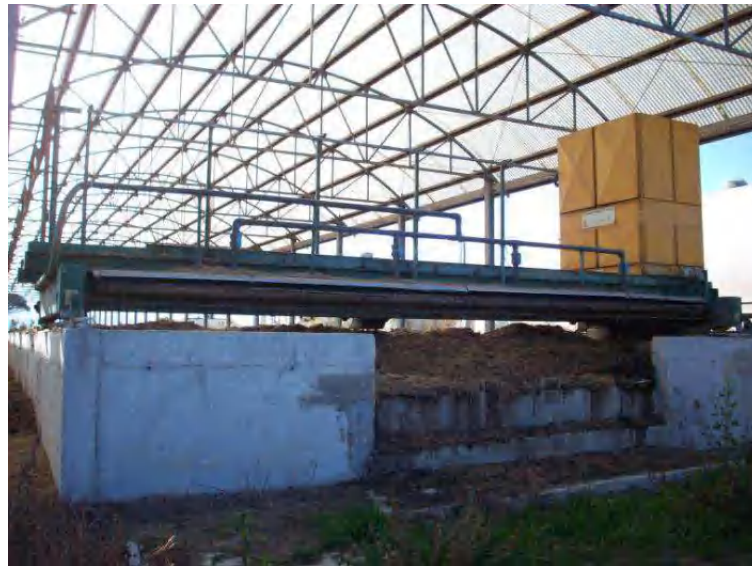
Fig. 1. Aerobic treatment facility.
