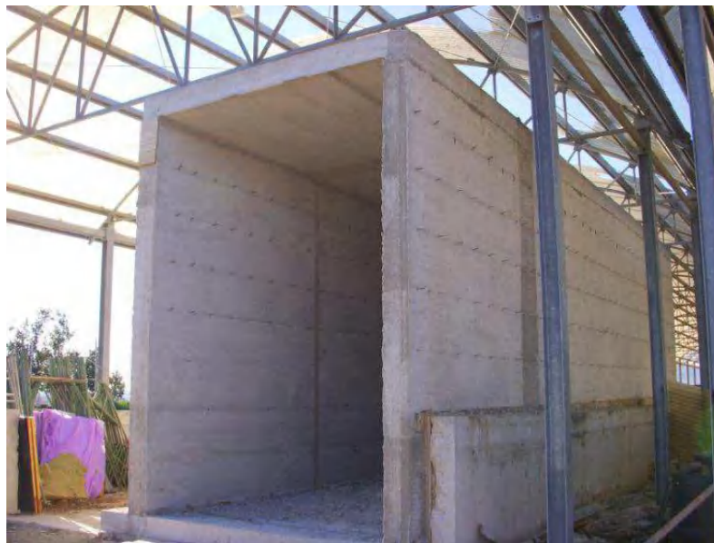
Fig. 2. SSAD cell during construction.
