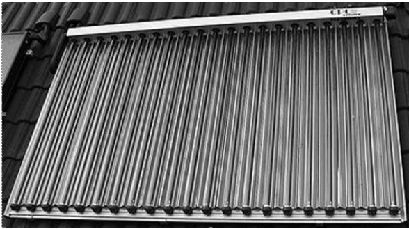
Figure 1 - Example of solar collector using an array of glass heat pipes.
