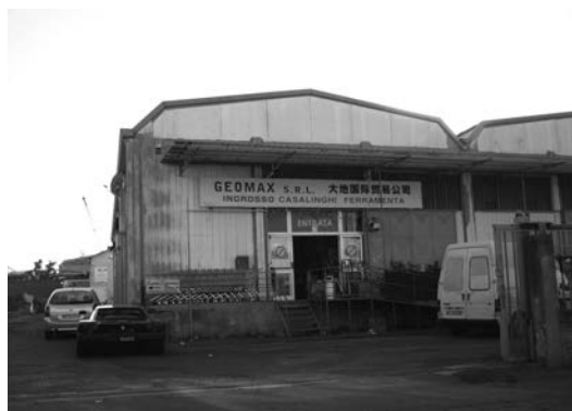
Fig. 6 - Storehouse in Via dell'Omo that allows free entry to VAT number owners
