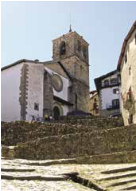
Fig. 6: Channels drains ( regaderas ) along the streets in Candelario, Spain (photo: M. Cadinu).
