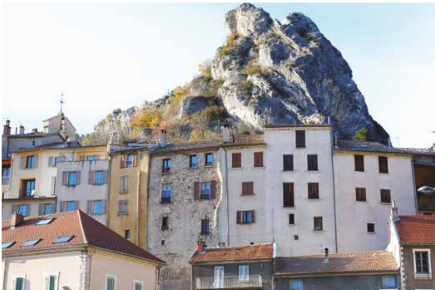
Fig. 5 Compact and grouped buildings; Serres in Upper-Alps department, France (photo: N. Sánchez).
