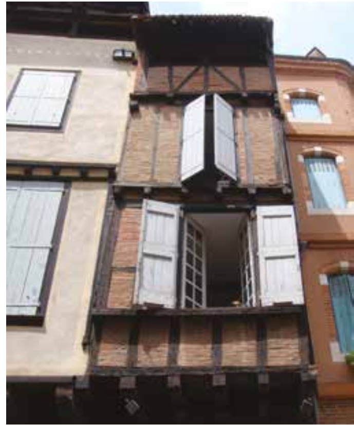
Fig. 17 External board and batten shutters in an old half-timber house at Albi, France.
