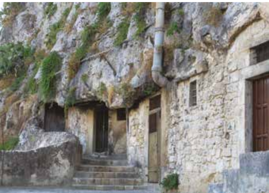
Fig.2 Underground dwellings in Scicli, Sicily, Italy.
