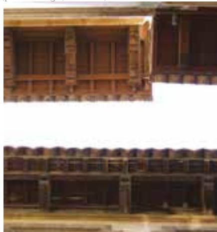
Fig. 1 Eaves in a street of Palma de Mallorca preventing the sun from impacting on façades and streets. Spain (photo: F. Vegas, C. Mileto).
