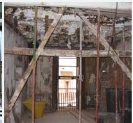
Old baraccata structure during restoration works site in Lamezia terme, Calabria, Italy (photo: E. Pelaia).
