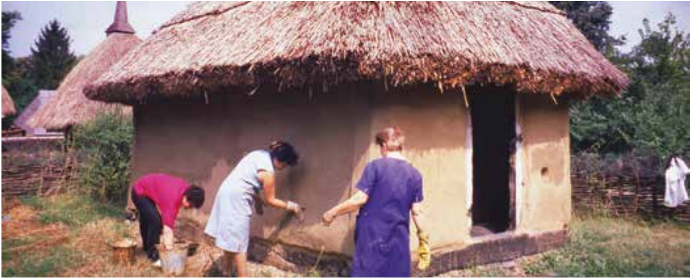
Fig. 12 Communitarian maintenance of vernacular buildings in Romania (photo: M. Correia).
