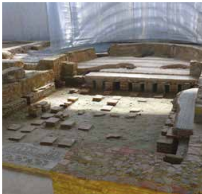
Fig. 2 Roman hypocaust. Villa La Olmeida at Pedroso de la Vega, Spain, II°-IV° centuries A.C. (photo: H. Guillaud).
