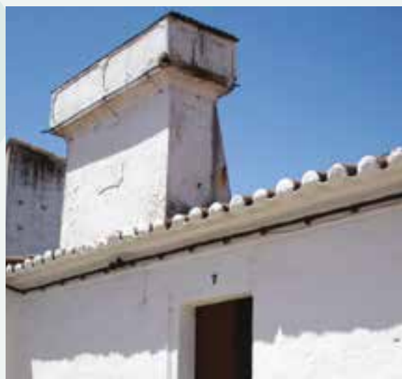
Dwellings in São Vicente e Ventosa: high thermal mass walls of stone and earth masonry (photos: I. Costa Carrapiço).
