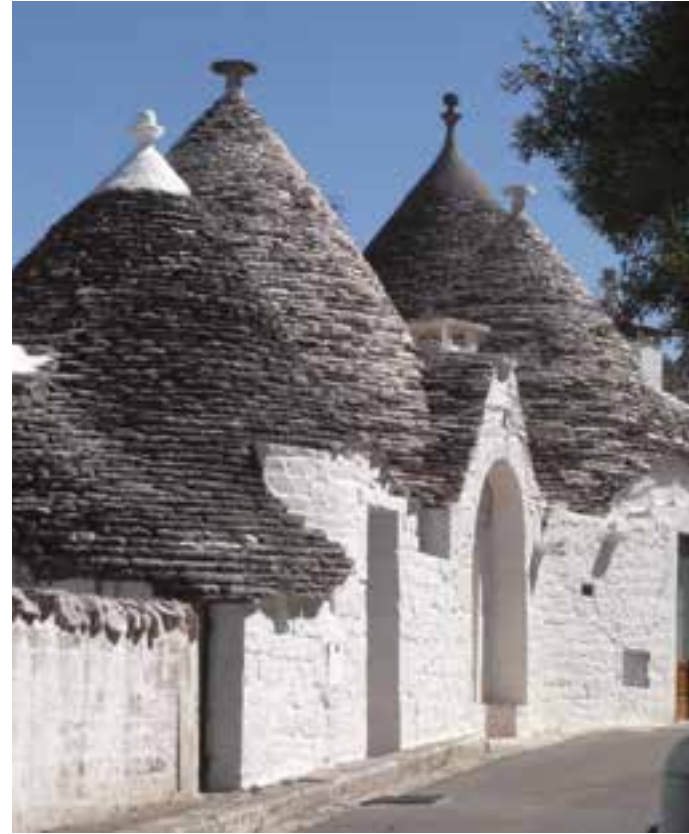
Fig. 3 Roof shapes and local materials. Trulli, Alberobello, Region of Apulia, Italy (photo: B. Özel).
