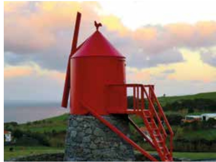
Fig. 8 Energy management: a windmill in the island of Faial, Azores, Portugal (photo: M. Correia).
