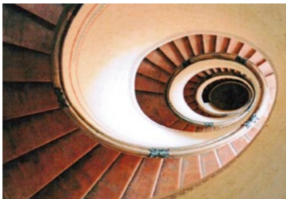
Fig.25. Palazzo Barozzi, the spiral staircase, ed.Visual Project
