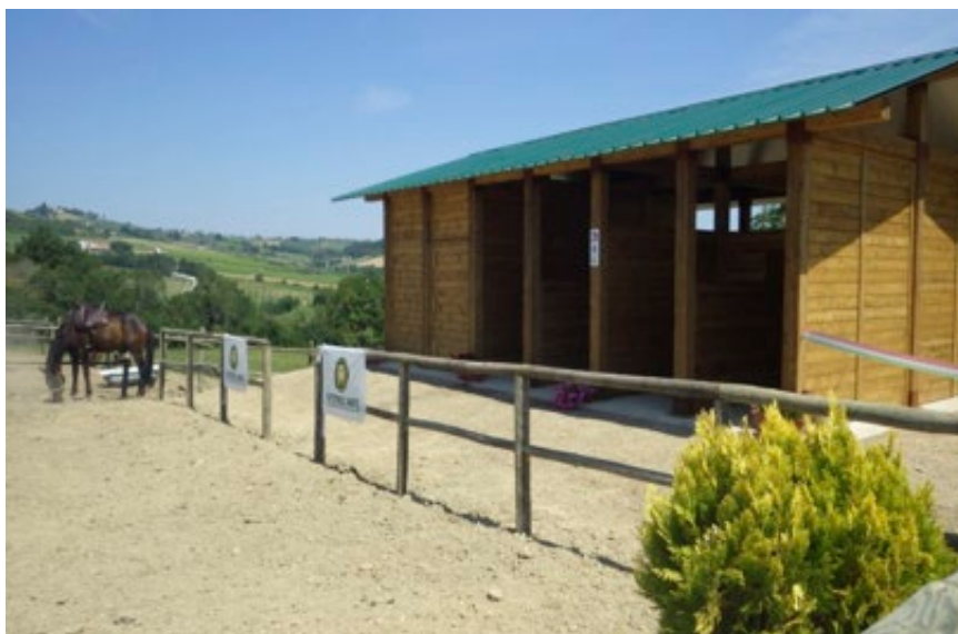
Fig. 6. Structure completed and inaugurated in June 2014
