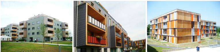
Fig. 1 Executed multi-storey wood-based residential buildings
