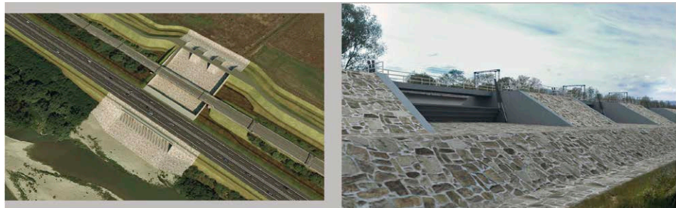
Fig. D-15. Side weir of the Pizziconi flood retention area (from www.gruppoeurostudio.it ).
