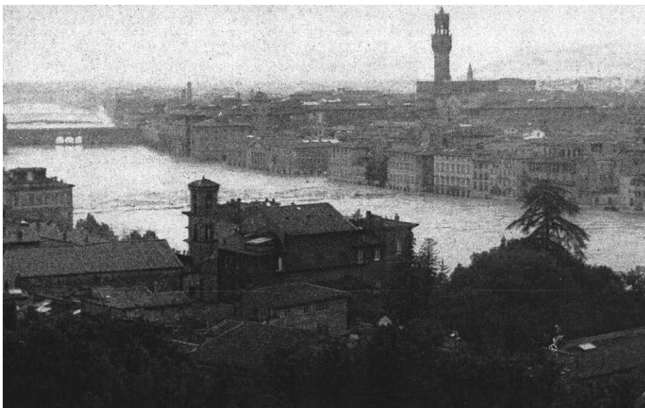
Fig. C-43. Overview of the Arno River showing Florence bridges during the 4 November 1966 flood: note in the foreground the Ponte alle Grazie that was completely submerged (Photo Caldini, reproduced from Principe and Sica, 1967).
