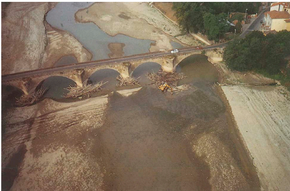
Fig. 3-9. The Buriano Bridge connects the banks of the Arno River along the Cassia Vetus, the old road which connected Rome to Florence, crossing Arezzo. It may possibly incorporate a preexisting Roman bridge. Buriano Bridge and Ponte Vecchio are the only historical bridges remaining along the course of the Arno River. The heightening of La Penna dam would lead to its submergence for less than 24 hours during exceptional floods (recurrence time of the order of a century) (Reproduced from 1996 Hydraulic Risk Plan).
