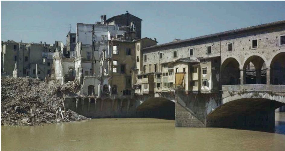
Fig. C-21. View of damage to the Ponte Vecchio from the east. The Germans destroyed all the bridges over the Arno River, with the only exception of the Ponte Vecchio, before evacuating Florence on August 11th 1944. The Ponte Vecchio was blocked by demolishing the houses at both ends and placing explosives on the bridge.
