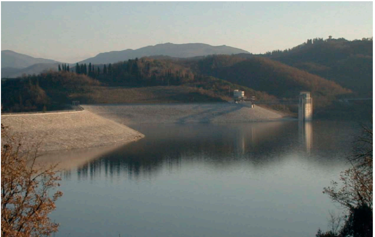
Fig. 3-11. The Bilancino earthfill dam in the upper Sieve basin (Photo reproduced from Caporali et al., 2005).
