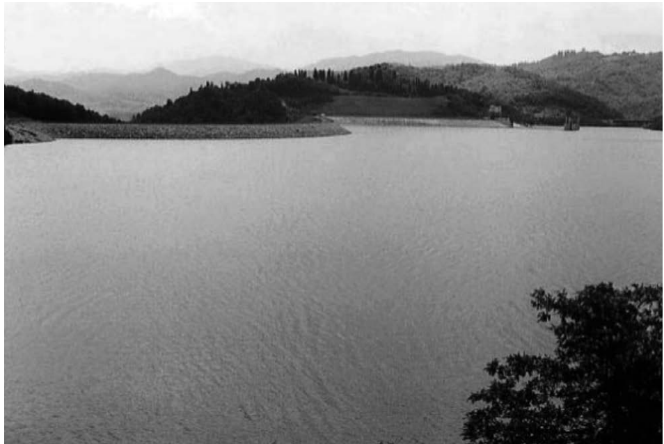
Fig. D-4. The Bilancino earthfill dam at the maximum storage (Courtesy by Dott. Grossi and Publiacqua).
