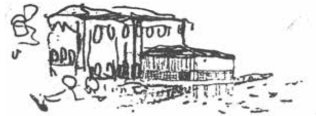
Le Corbusier's journey into the East. Stambul panorama from Eyup and wooden houses on the Bosphorus
