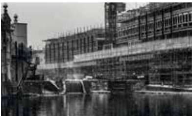
Figure 5. Lock and Building in Progress
