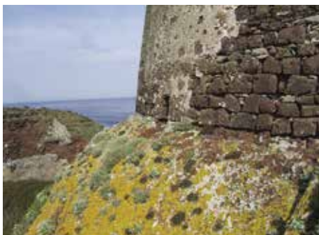
Figure 2 – Tower of Zenòbito: rock basement and residues of plaster.
