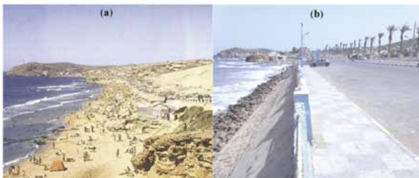
Photo 3 – Difference in the state of the Bomo beach: (a) Bomo beach in the 1980s: a wide beach supplied by the aeolian effects of the foredune behind the wilaya road No. 84. (b) Bomo beach in July 2017: fixing the foredune by reforestation and establishment of a rockfill to protecting the road for wave action. (Photo credit: A. Bougherira).
