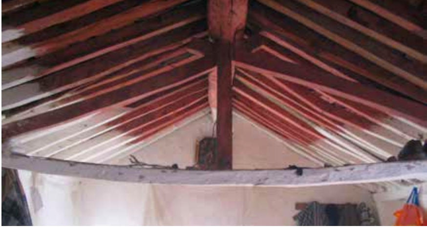
→ Berber timber roof (R2a) Interbal view
