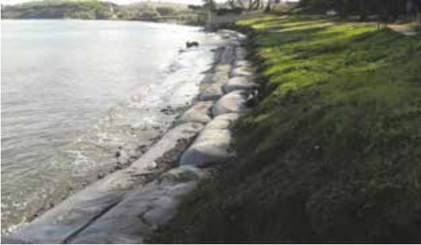
Figure 5 - Sacks of geotextile cloth containing sand.
