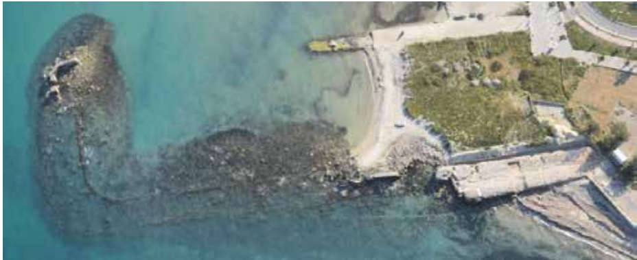
Figure 3 - San Cataldo (Lecce, Italy): Roman and 20th-century piers ruins aerial view (LabTAF, 2013).
