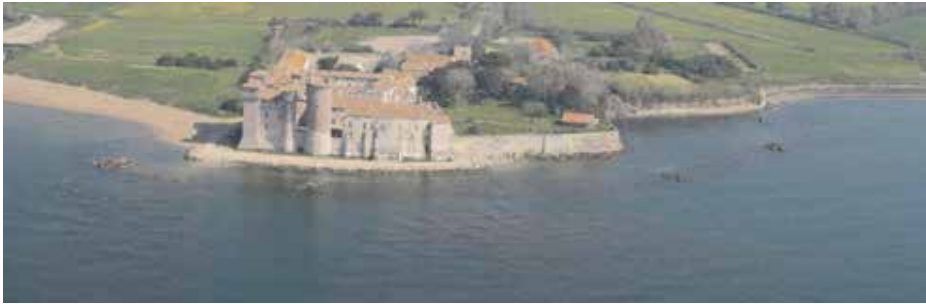
Figure 7 - Some other structures just under the surface of the sea, on the east corner of the castle.
