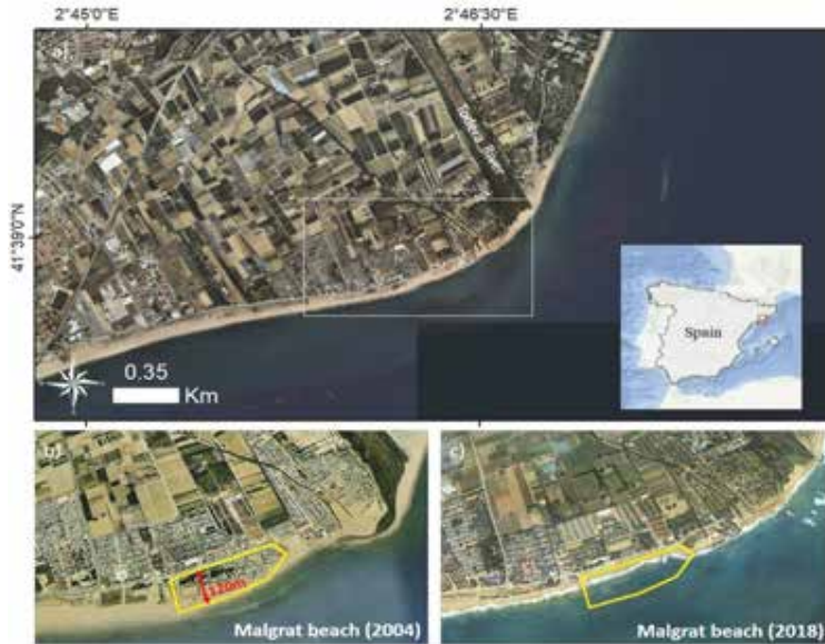
Figure 1 - Location of the study case site (a), Malgrat beach (Spain) and situation of the coast in 2004 (b) and 2018 (c). The yellow polygon indicates the coastal area lost due to erosion problems along the 14 years.
