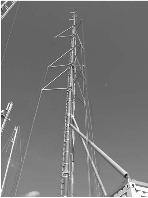
Figure 7.1 View of the cable stayed mast with the truss systems and the two pipe rods.
