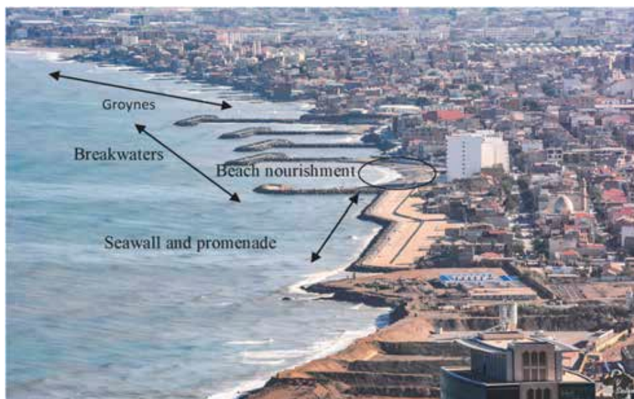
Figure 9 - Illustration of protective structures at the study site (Photo taken by a drone in 2019, Credits: Anonymous).
