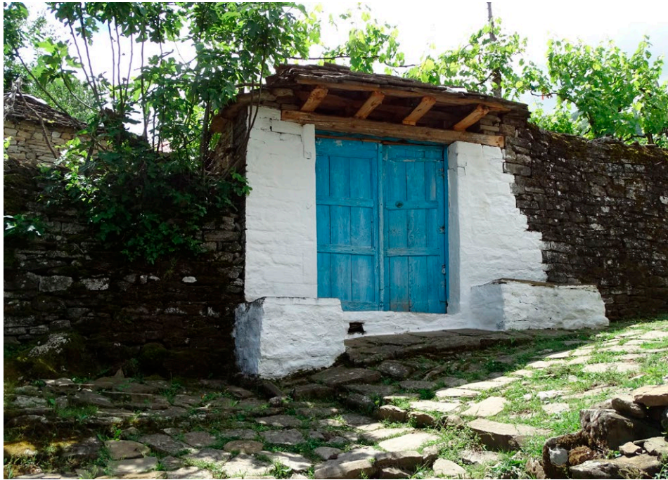
Figure I-4.3.2 A traditional entrance door to a courtyard with the sofat .
