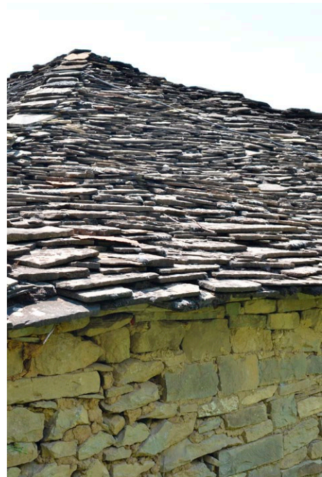
Figure I-2.7 – Leusë. A traditional roof covering made of dry-assembled stone slabs.
