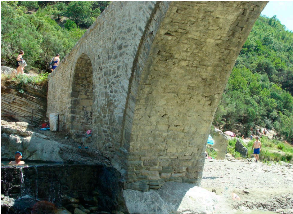
Figure I-5.1.7 – A view of the bridge looking upstream showing the restoration work carried out in 2018.
