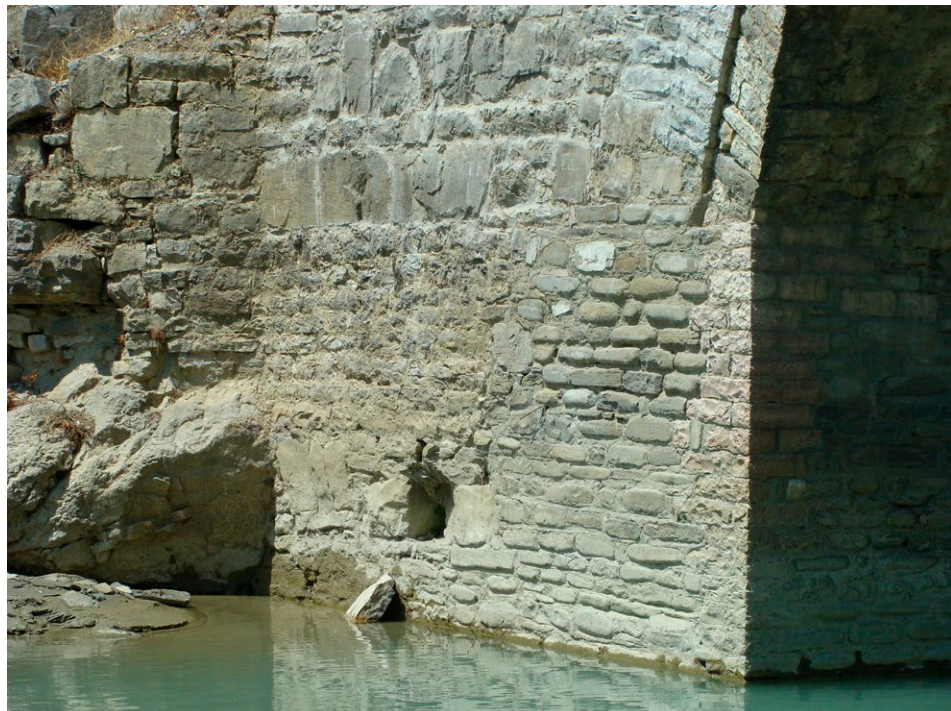
Figure I-5.1.6 – A detail of the abutment restored in 1982.
