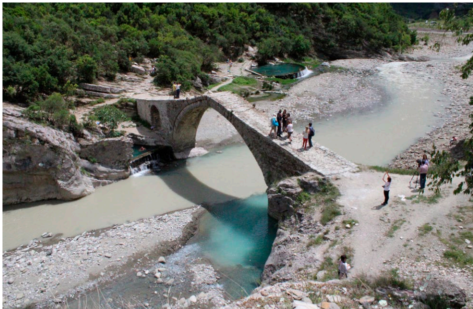
Figure I-5.1.3 View of the Katiu Bridge and of the thermal baths.
