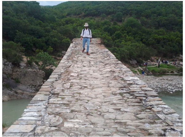
Figure I-5.1.4 – The roadway of the bridge.
