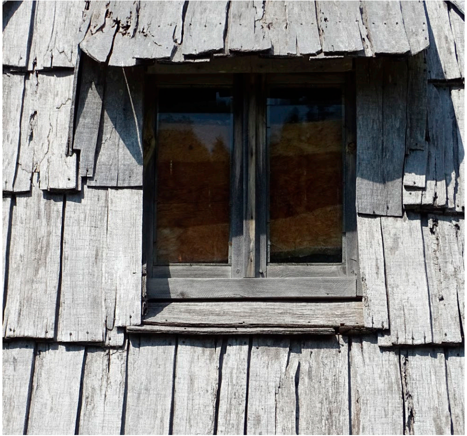
Figure II-2.8 Detail of a mountain hut roof, covered with wooden shingles.
