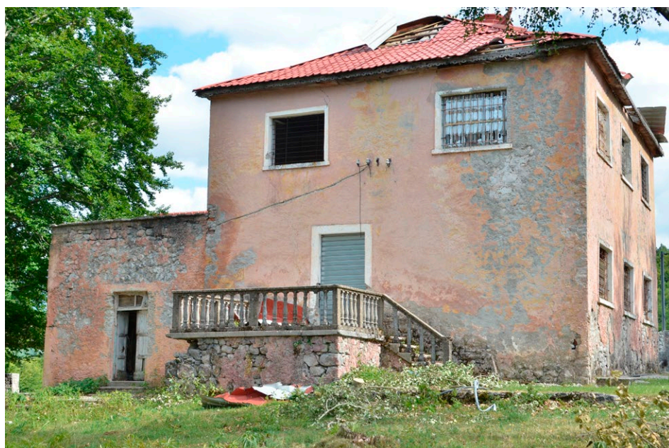
Figure II-5.4 Above: A one-storey villa with a half-hipped roof. Below: A two-storey villa with a hipped roof.
