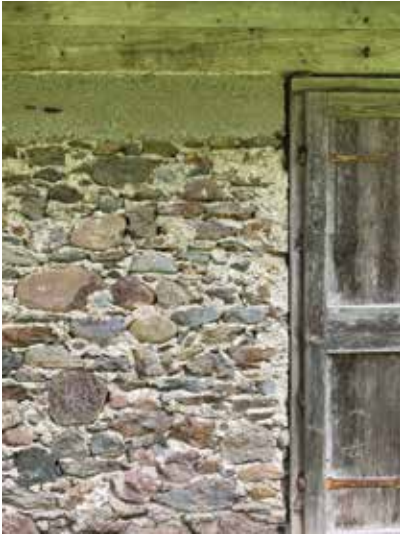
↑ Fig. 5 Detail of the external walls of a traditional rural building "tabià" in Dosoleudo (Comelico Superiore). (photo by C. Valiante, 2020).
