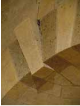
Fig. 6 Vulnerability A4: The southern minor apse: rotation of the keystone.
