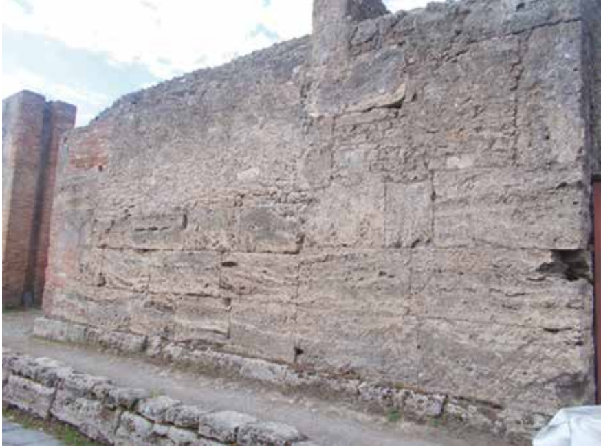
Fig. 5 Opus quadratum characterizes the walls of Vesonio Primo's House.
