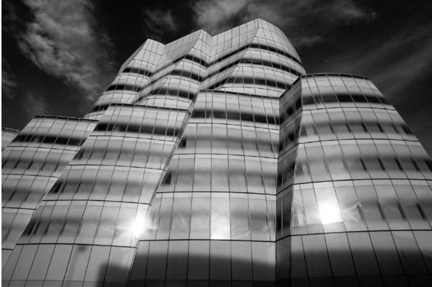
Fig. 3 – Frank Gehry, IAC building New York City, 2007-2008
