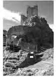
VIEW OVER THE TOWER
